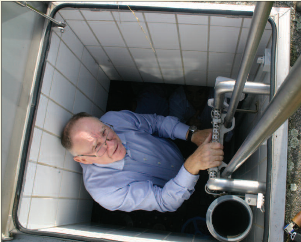
NFGWS Chairperson, Brendan O'Mahony enters a chamber that collects water from several springs for distribution by the community-owned drinking supply of Gramastetten in Upper Austria. See report on pages 15-18.
